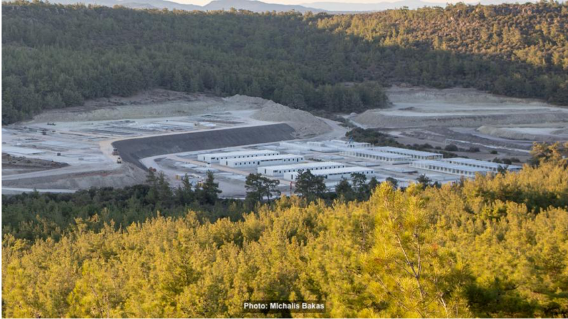
The under construction new CCAC in the Vastria region
